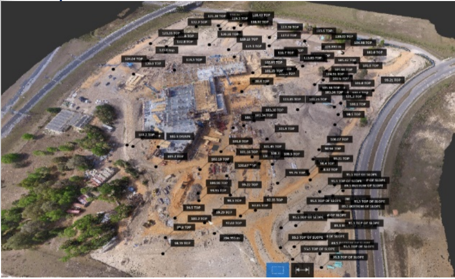
Aerial photography during the construction
